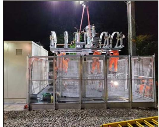
Fig. 1: Lifting the base frame structure
