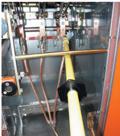
Pic. 12: Mounting of a earthing and short-circuiting device with a earthing stick
