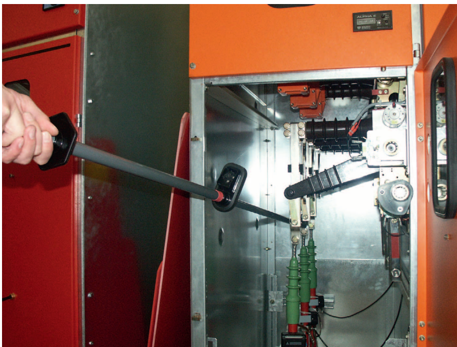
Pic. 8: Passive voltage detector with optically LED-indicator
