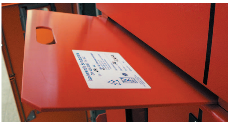
Pic. 14: Inserting of a protective barrier
