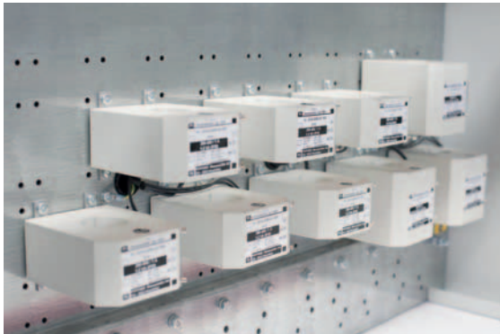
Current transformer installation
