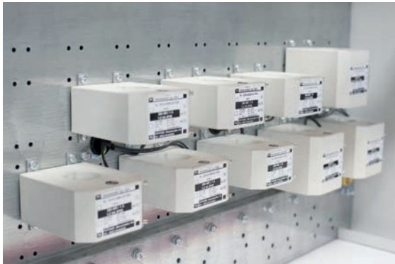
Current transformer installation
