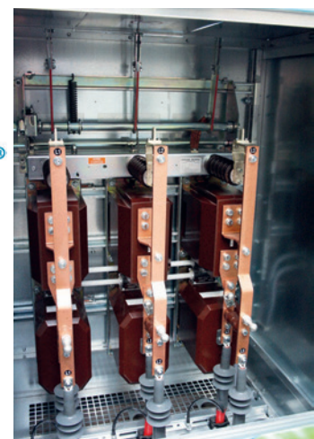
Fig.: Measuring panel W12/24 with arc-fault protection limiter ABS®
