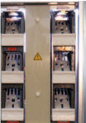
Pic 5: Busbar insulating cover
