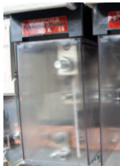
Pic 6: Cable insulating cover
