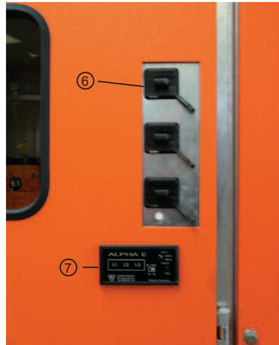
Picture: Capacitive interface and short-circuit indicator
